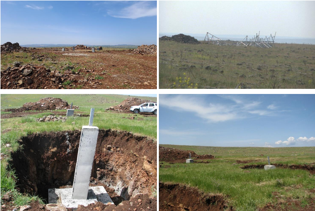
Figure 3-1: Photos of General Site Activities (Dated May 10, 2023, taken by WSP Golder)
