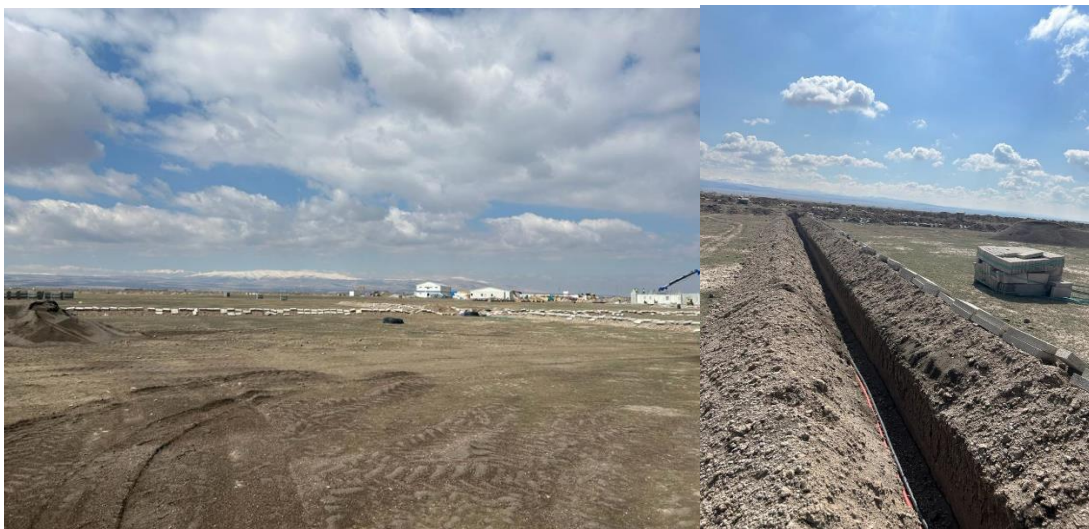
Figure 3-2: Photos of General Site Activities (Dated March 21, 2023, taken by WSP Golder)
