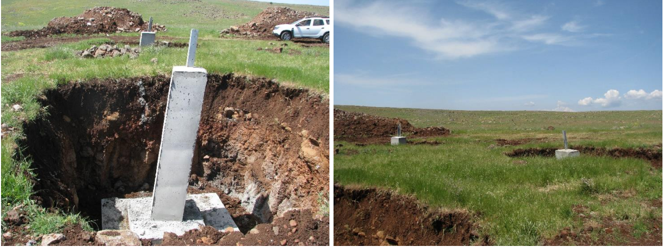
Figure 2: Photos of General Site (Dated May 10, 2023, taken by WSP)
