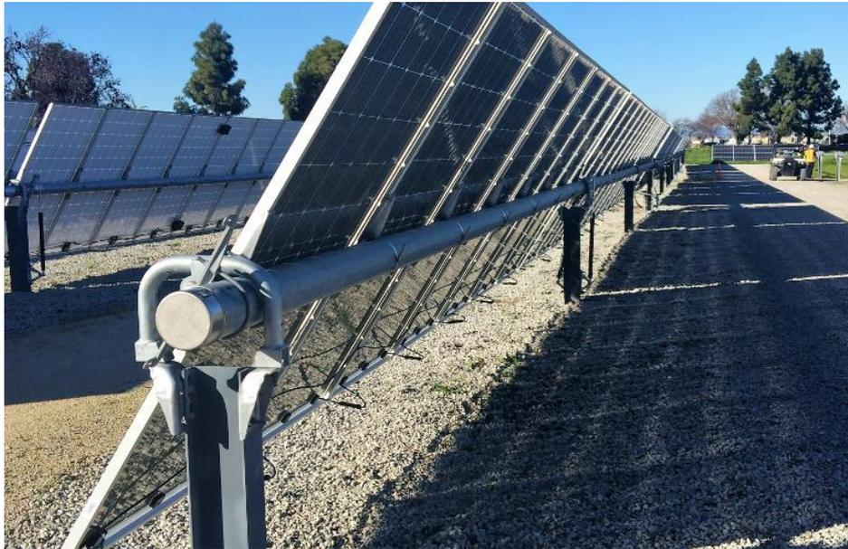
**Figure 2-6: Single Axis Tracker System in Combination with Bi-facial Modules<sup>1</sup>**
