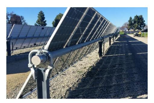
Figure 2-6: Single Axis Tracker System in Combination with Bi-facial Modules<sup>1</sup>
